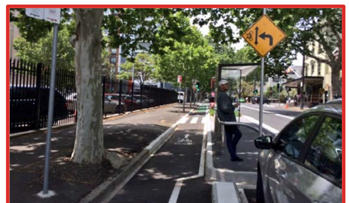
Image 3 Campbell Street in Sydney shows ideal separated cycleway infrastructure with a bus stop and pedestrian refuge. (Sarah Stace)
