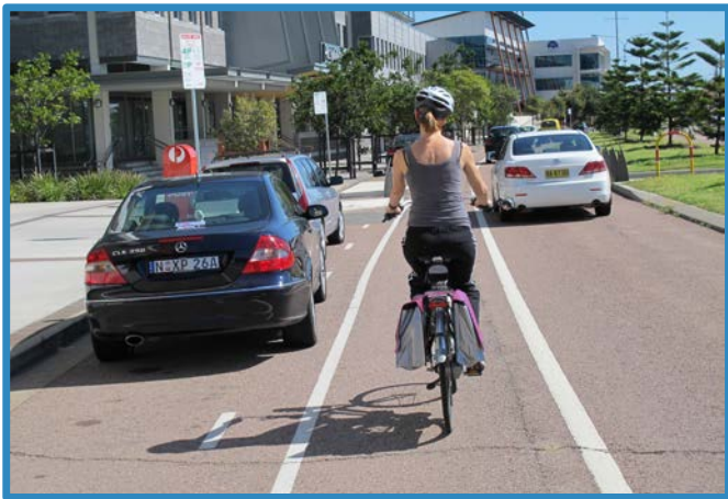
Image 17 Honeysuckle drive cycleway on road with minimal buffer and still in car door lane. (Bernard Hockings)
